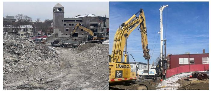
NOTE: Demolition is paused while the demo debris is processed, sorted and trucked out.
